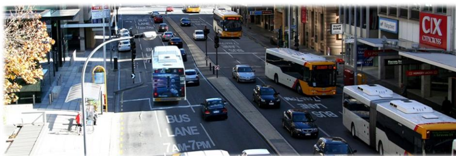
DIT: Priority bus lane project
